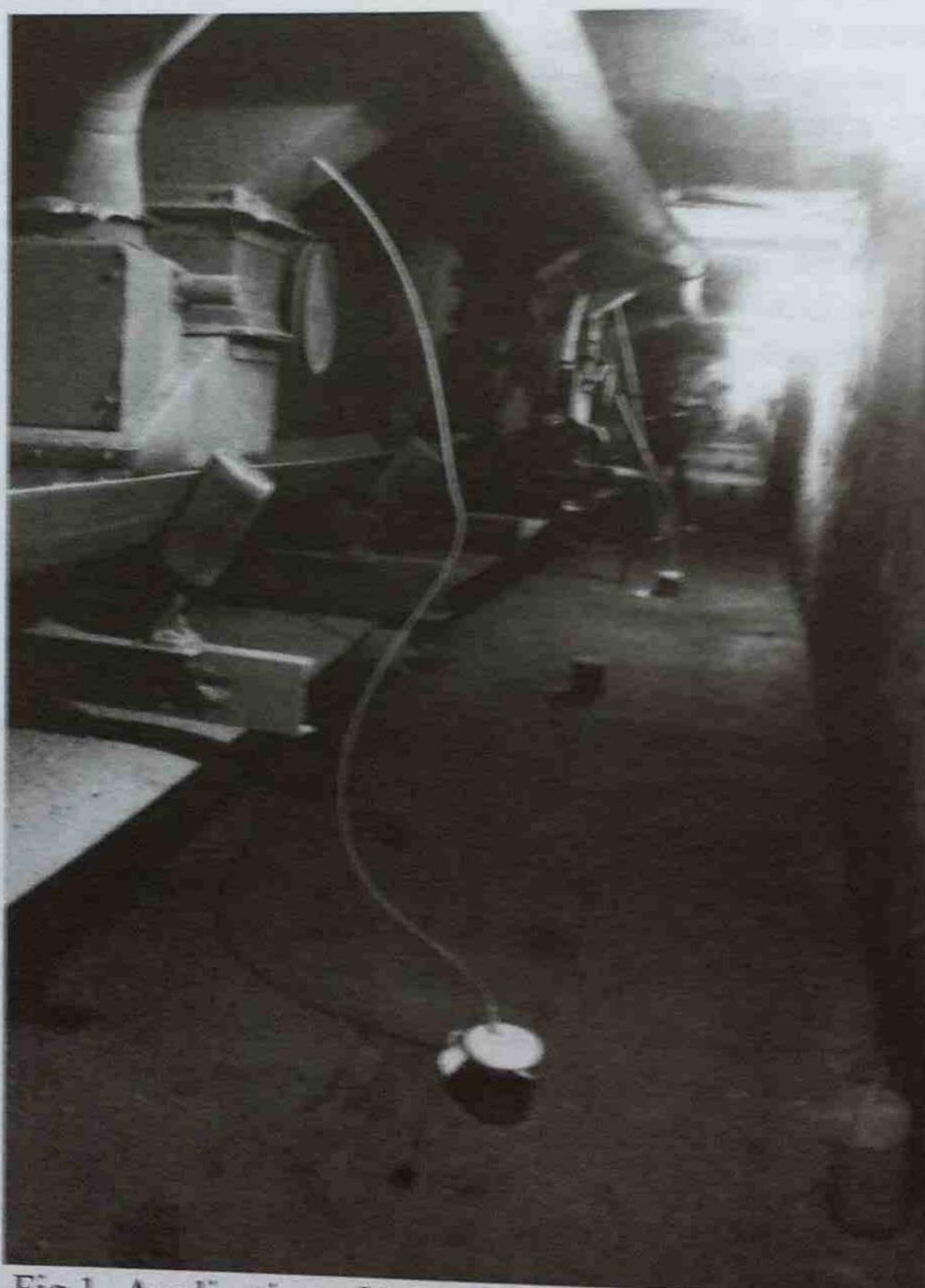
Fig.1- Application of SGF-M2 generators to silo bins
